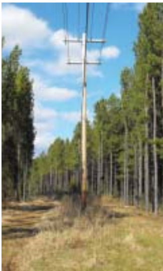
Continued maintenance of our right-of-way corridors decreases outages.
