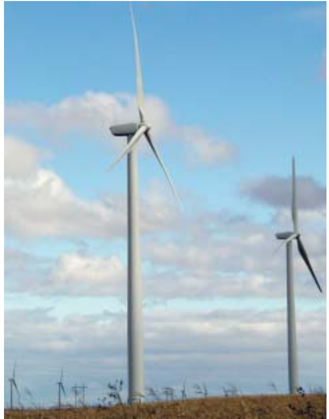
The Story County Wind Energy Center, located near Colo, Iowa consists of 100 wind turbines, each capable of producing 1.5 megawatts of wind power.
